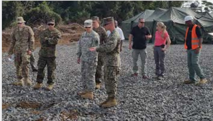
Michaella Olson talks with Navy Seabee engineers during a visit to an Ebola treatment unit construction site in Sinje, Liberia. The ETUs were built during Operation United Assistance, the Defense Department operation supporting the U.S. Agency for International Development-led humanitarian effort to contain the spread of the Ebola virus in West Africa.
